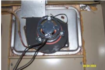
virtually eliminating the potential for fumes to pass through a crack in the heat exchanger into the flow of house air. However, the inducer fan creates the potential for a different hazard.
