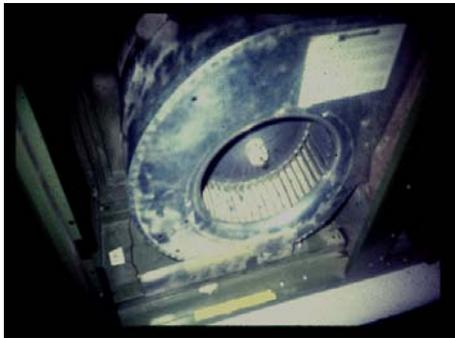
of supply and return ducts. The blower fan is typically located in the blower housing *upstream* of the heat exchanger. It draws air from the house, through the return duct, and then pushes it across the heat exchanger and through the supply ducts to the living spaces. In this typical configuration, the return duct is under negative pressure and the supply ducts are under positive pressure. Air will be drawn in through openings in the return and blown out through openings in the supply. By
