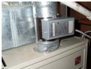
An early energy efficiency improvement addressed house air lost up the flue between cycles. A simple solution was the *vent damper*. Installed on the vent connector, this heat activated damper opens when the system is running and closes when the system is at rest. Electronic vent dampers have an electric motor that opens and closes the damper. A malfunctioning vent damper is likely to cause a back draft.
