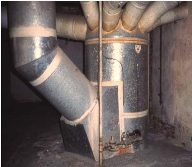
the outside of the combustion chamber. Air falls in the return because it is cooler and therefore heavier than the warm air that is rising through the supply ducts. Because the distribution medium is air and distribution is accomplished by simply allowing the warm air to rise naturally through the supply ducts, we call this appliance a gravity furnace.
