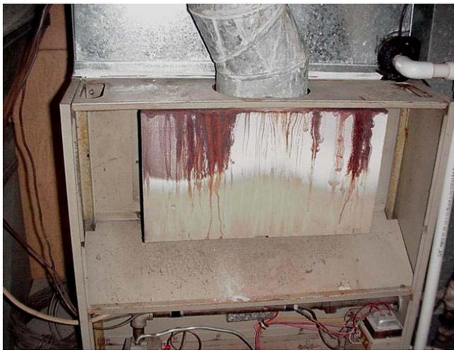
With the system drafting properly, air is drawn in through the draft hood diluting the combustion fumes. The water in the fumes remains a vapor and is suspended in the flue gases. If however, the system begins to back draft, flow reverses, and water condenses. Water in the steel vent connector or at the draft hood can promote rust. Water condenses, evaporates away, and leaves residual mineral deposits behind. Rust on the vent connector or in the draft hood is evidence of back draft.
