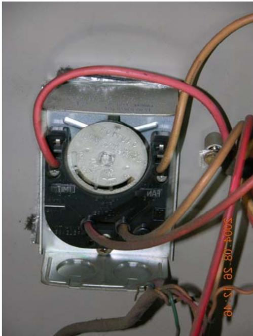
There is a third set-point on the fan/limit switch. This is the high limit. The fan on set-point determines the temperature at which the fan turns on. The fan off set-point
