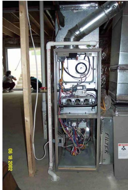
There is potential for a small leak in a burner to allow gas to build up in the heat exchanger between cycles. If the gas concentrations in the heat exchanger reach the flash point prior to ignition, it is possible that the igniter might ignite this gas and cause an explosion. In order to circumvent this possibility, the inducer fan must perform a purge cycle prior to ignition. The startup sequence for an induced draft system is slightly different from our conventional furnace:
