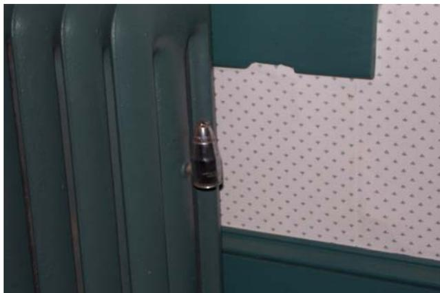
Heat is distributed through the living spaces in a convective loop. The steam being cooled condenses back to water releasing the latent heat.
